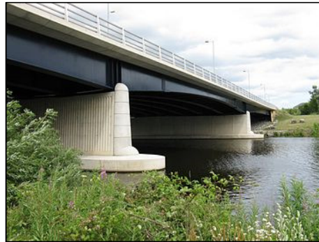
Photos 15, 16, and 17: High Quality Concrete finishes on bridge piers
