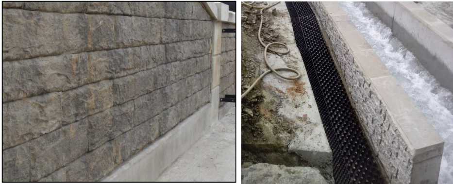
Photos 11 and 12: Pigmented Concrete with masonry imprint (Derwent Water and Linguen Weir)
