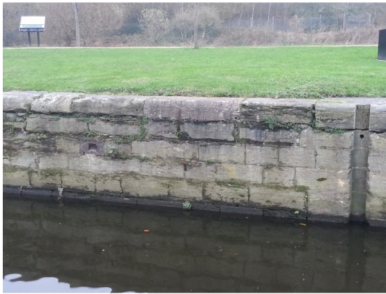
Photo 7: Typical material along Knostrop Cut
