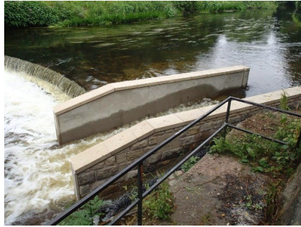
Photos 9 and 10: masonry cladding at Burley Mill Fishpass
