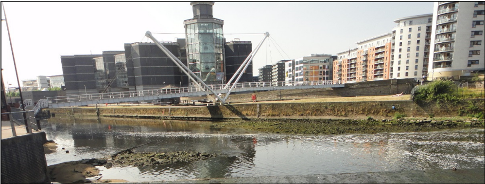
Photo 5: Buildings on the right bank – Clarence Dock, Royal Armouries
