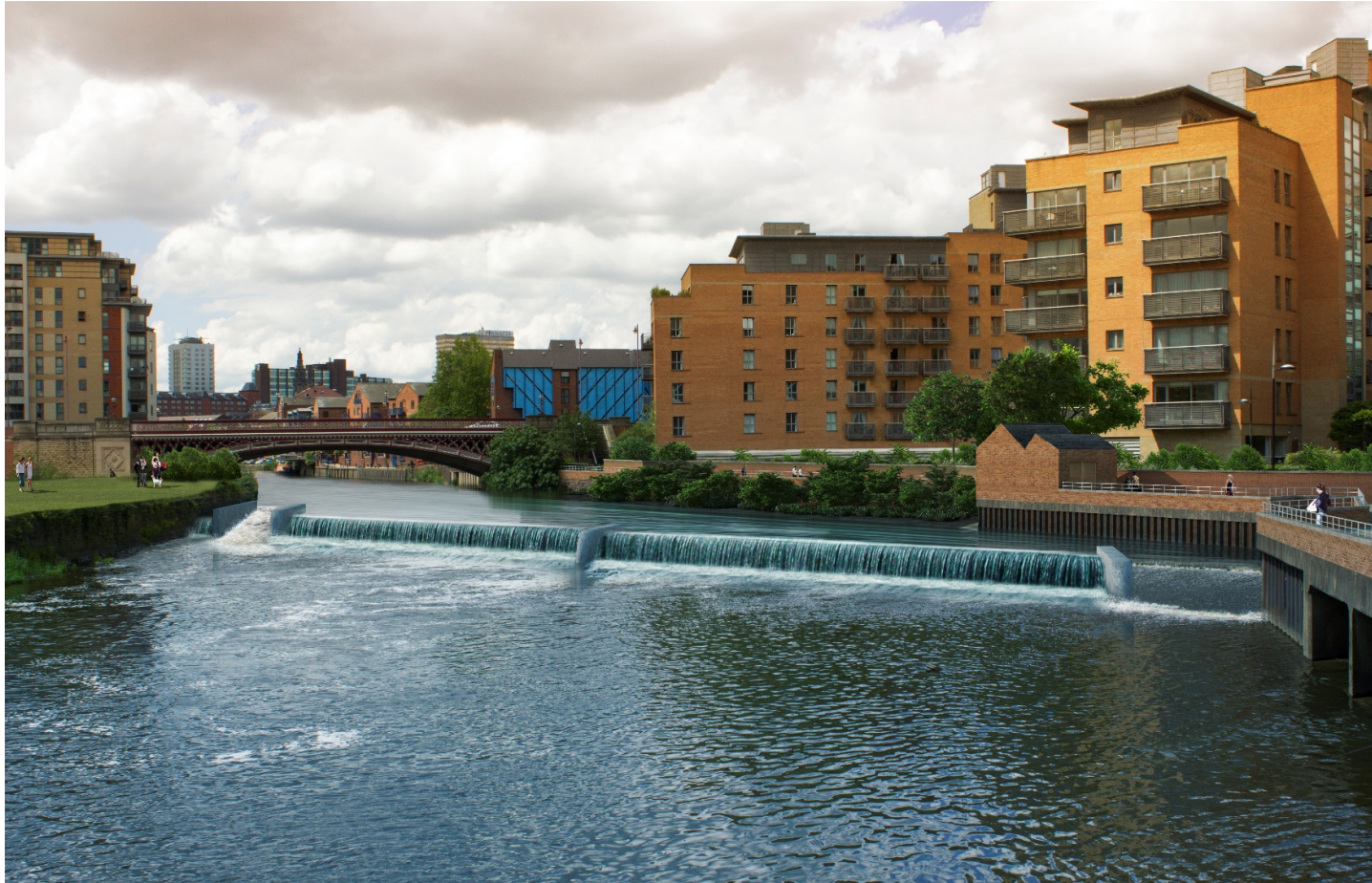
Figure 7: Downstream visual representations of Concrete finishes
