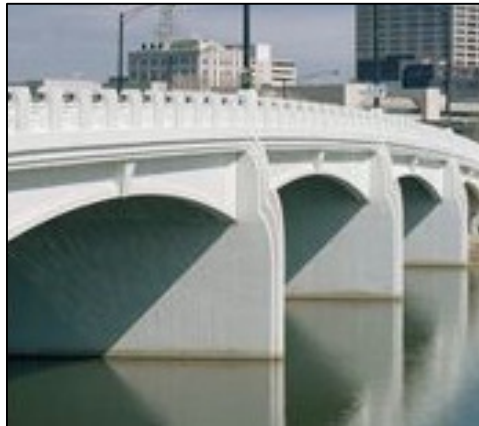
Photos 15, 16, and 17: High Quality Concrete finishes on bridge piers
