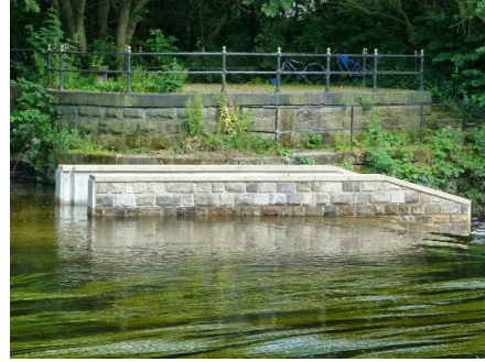
Photos 9 and 10: masonry cladding at Burley Mill Fishpass
