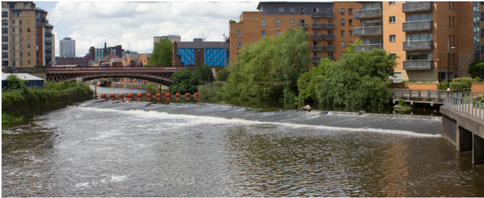
Photo1 - Existing walls around Crown Point Weir have various finishes.
