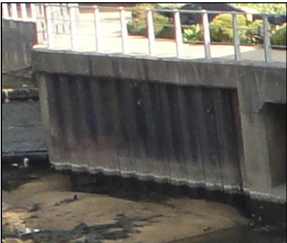
Photo 2: Fearn's Island River Wall, adjacent to weir Photo 3: Turlow Court River wall, adjacent to weir Photo 4: Fearn's Wharf River Wall
